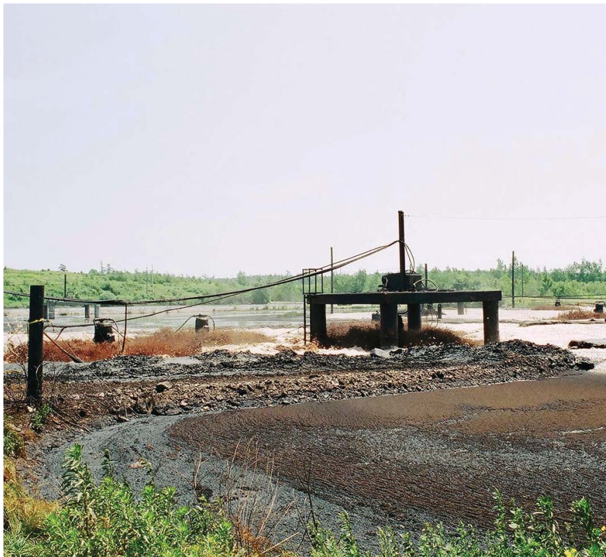
Biosolids Storage Lagoon
