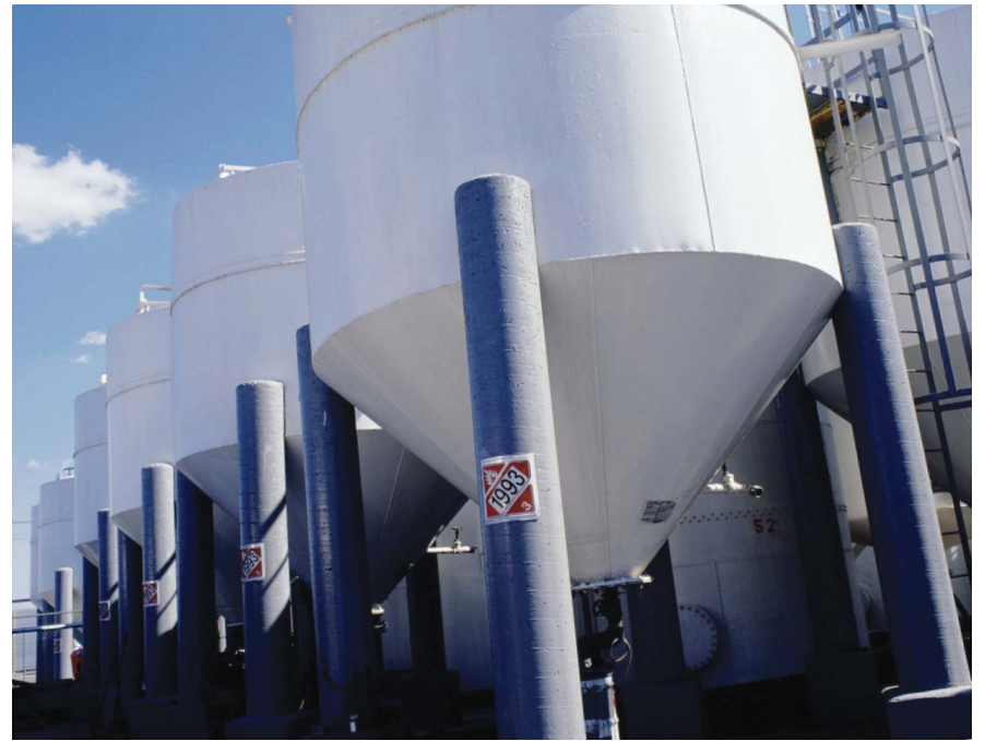
Fielding's recycling plant.
