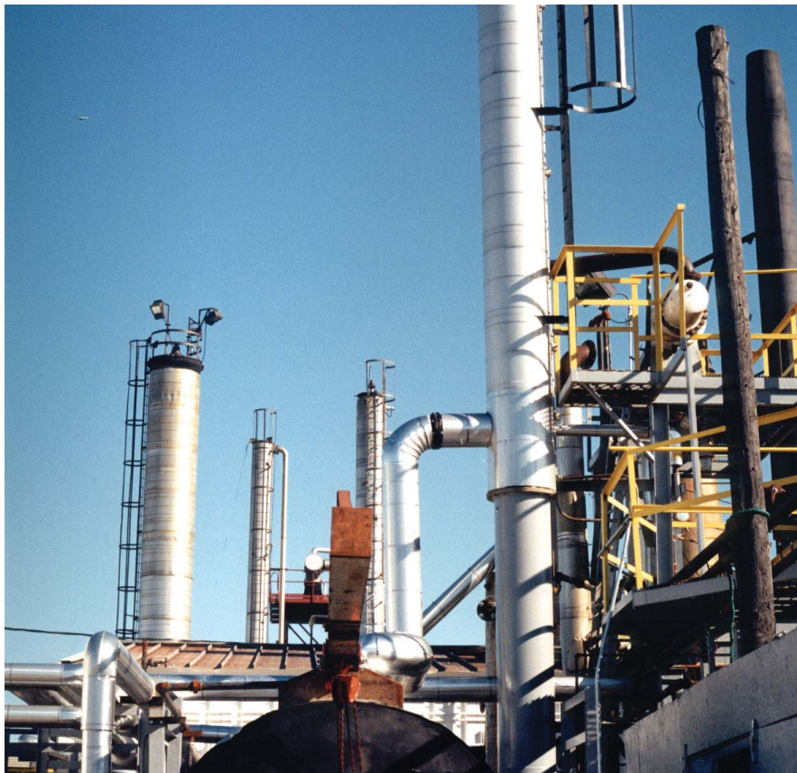
Fielding's recycling plant.
