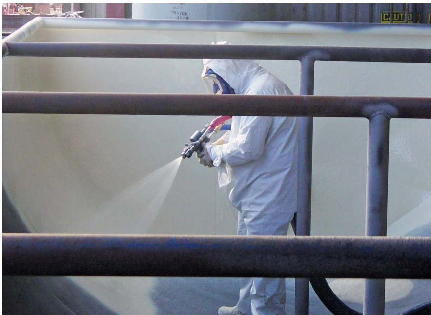
Spraying Rhino Linings' Hi-Chem 11-70 into a frac tank.
