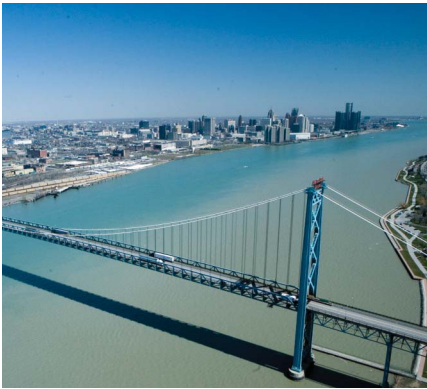
Still the only bridge in town ... the Ambassador Bridge links Detroit and Windsor, ON.
