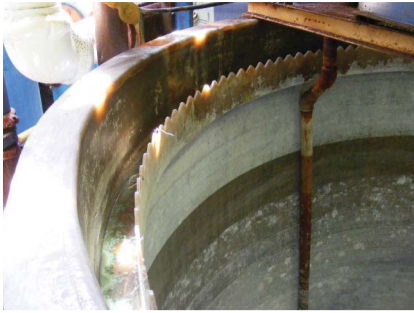
Empty circular clarifier.
