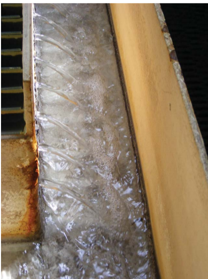
Clarifier effluent shows the top clear water with solids (sludge) removed.
