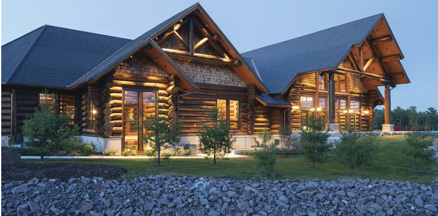
The 34,000-square foot Canada House at Killarney Mountain Lodge is currently the largest log conference center in the world. It was protected inside and out with Sansin Classic 1-2-3.
