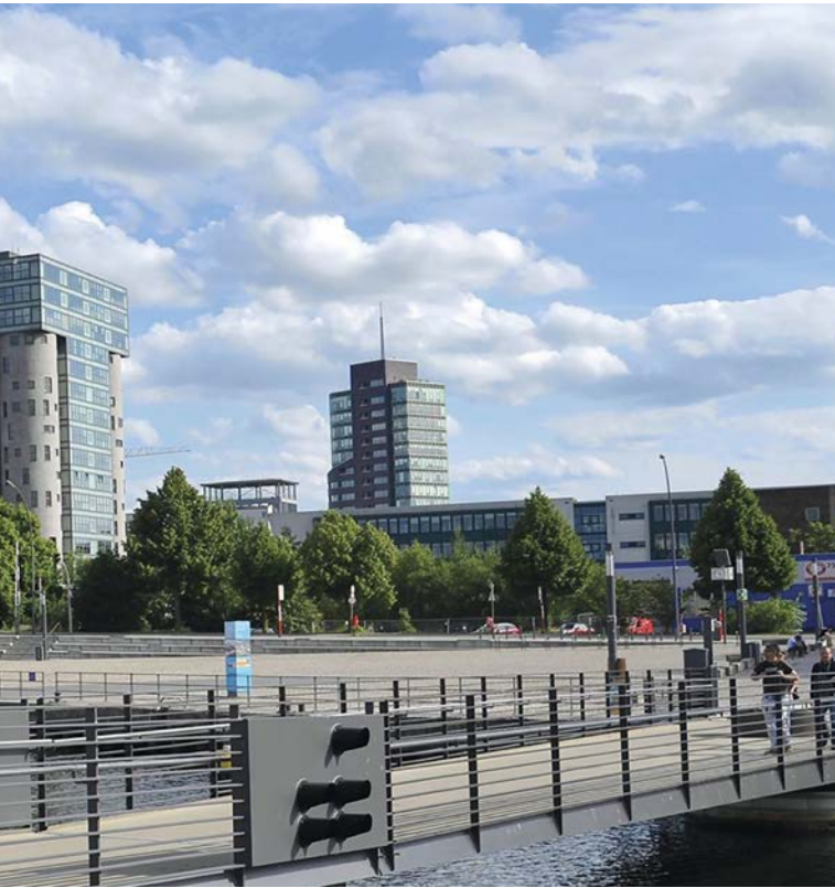
The Hamburg Bridge after treatment.
