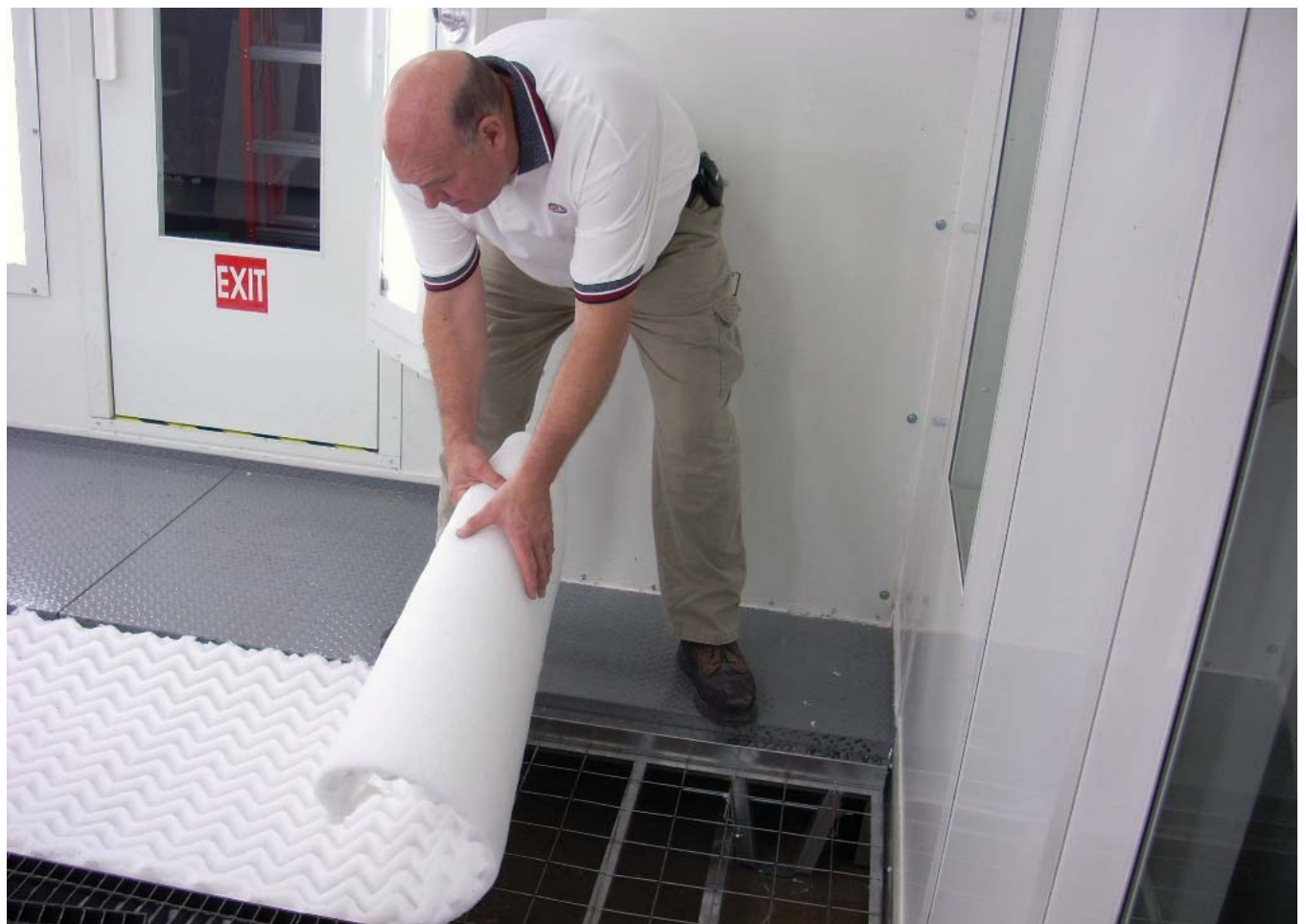
Installing the GFSWAVE spray booth filter media.
