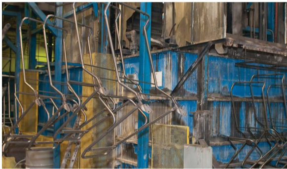
Shopping Cart Chassis traversing along E-Coat line overhead conveyor.
