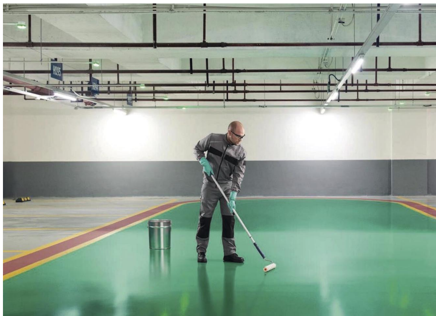
Applying a Covestro Pasquick coating to an institutional floor.
