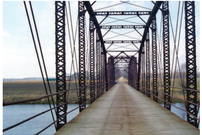
Iron-supported bridge in Woolwich Township, ON. Photo: Woolwich Twp.
