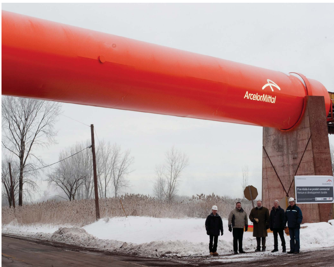
Ferrinov pigments were used in the coating formulation for this large overhead structure housing a conveyor system in Quebec. See story in the news section of this issue of CFCM.
