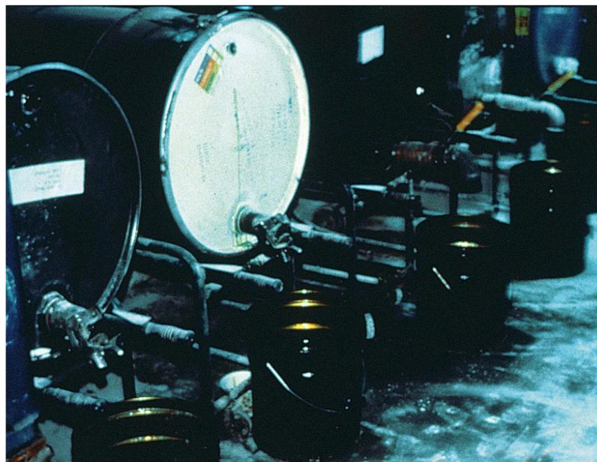
Drip buckets should not be used as chemical additive transfer buckets. Keep the area clean and dry.
