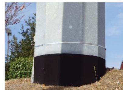
Chemline Incorporated announced the immediate availability of its spray-applied coatings specifically engineered for the corrosion protection of galvanized steel poles and structures: Chemthane 2261. The 100 per cent solids, (Zero VOC) fast cure coating is applied in a single coat, multi-pass technique directly to a prepared substrate. No primer is required.
